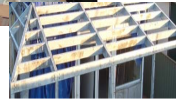
Roof structure as kitset
